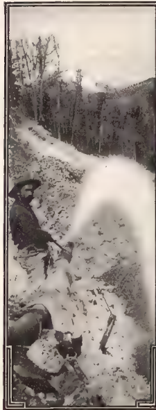
Caswells Piping the Decomposed Porphyry on the Surface of their Mine
